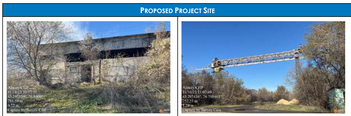
Figure 2-4 General Photos of the Proposed Project site
